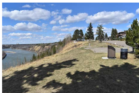
The landslide's location has become a popular lookout over the North Saskatchewan River.
