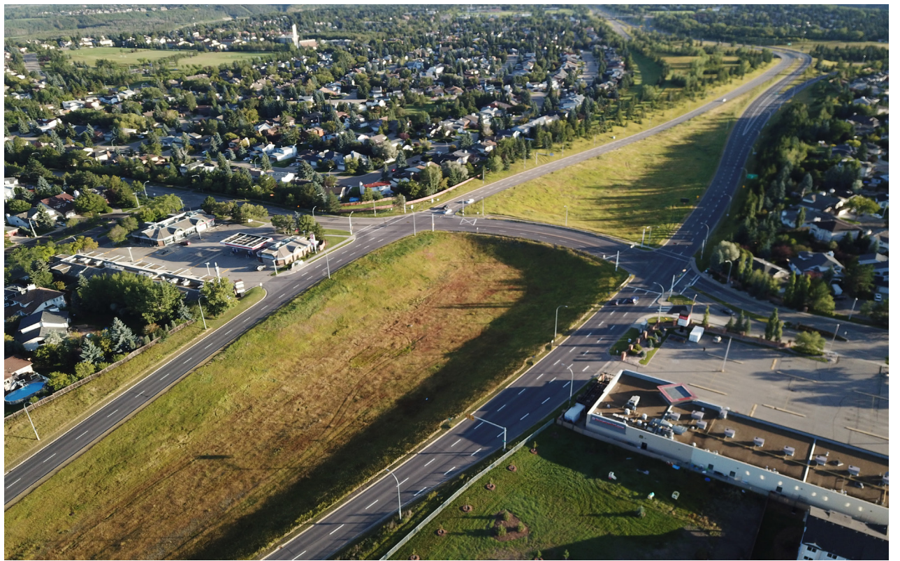
The intersection of Terwillegar Drive and 40th Ave., seen here (looking North), is one of four intersections that will see the addition of "smart signalling" technology to ease traffic flow
