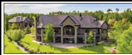
Rural Parkland County $5,700,000 Custom built executive estate. 6941 sq ft walkout bungalow on 2.5 acres. Incredible. ML# E4149615
