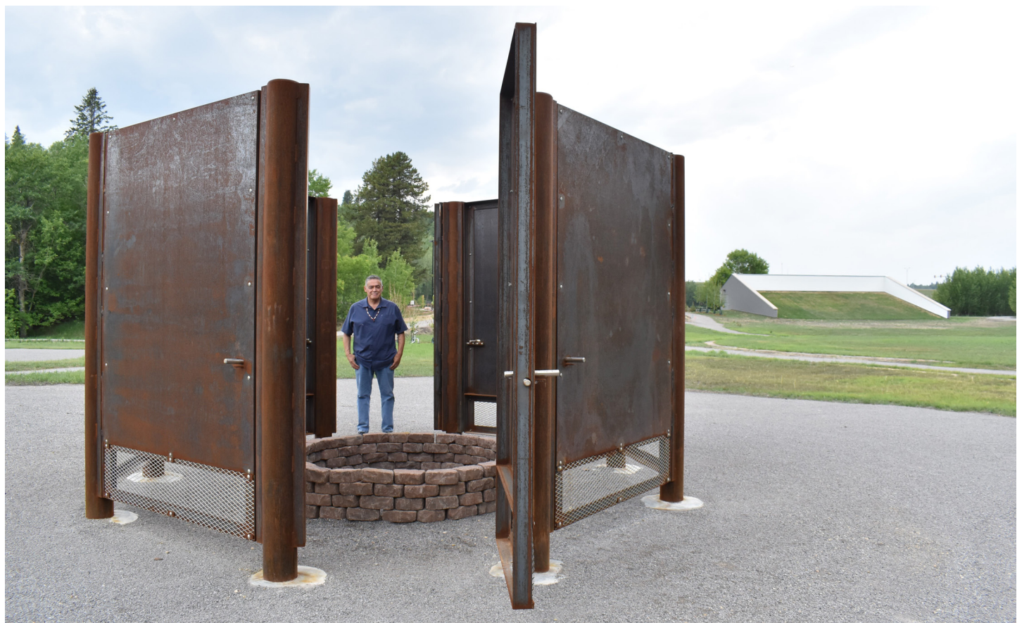
Project manager Lewis Cardinal stands by a fire pit that will be used to heat stones for sweat lodges. The doors around the fire-department-required enclosures are designed so participants can face whichever direction the ceremony requires.
