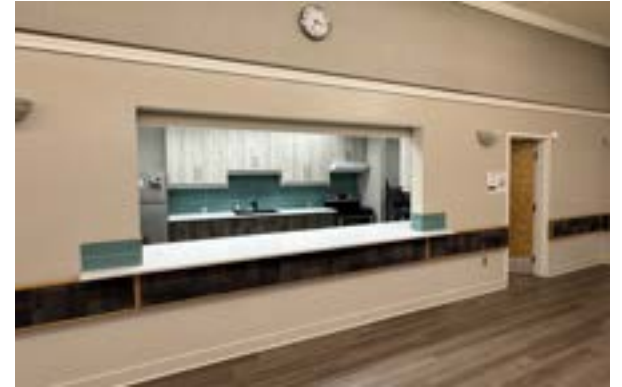
The renovated kitchen at Brookside Hall is ready to go, once again able to host your gathering. Find hall-rental options at riverbendonline.ca .
