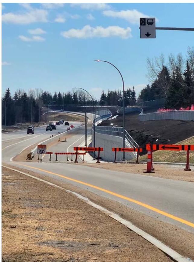
A newly constructed bus-only lane connects 53rd Avenue to Terwillegar Drive in Riverbend, part of a broader road expansion project aimed at improving transit flow.
