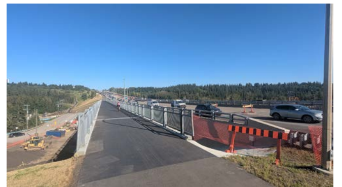
The new Rainbow Valley Pedestrian Bridge provides a broad route for cyclists, pedestrians and other active-mobility users over Whitemud Creek.
