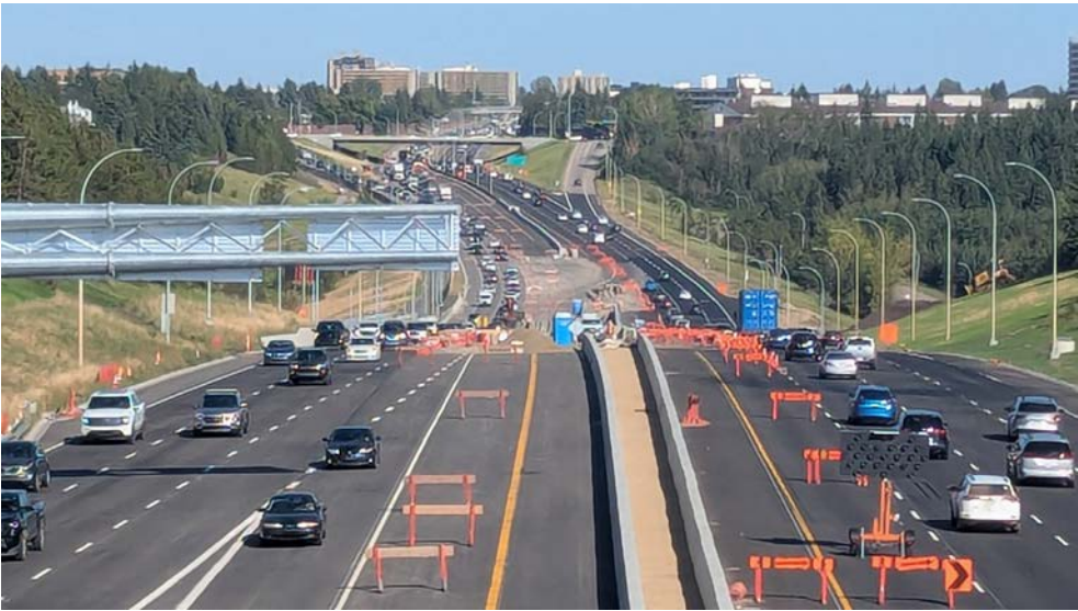
The Rainbow Valley Bridge is now open as part of Stage 2 of the Terwillegar Drive Expansion project, with remaining work on Whitemud Drive expected to wrap up this fall. Photo: Michael Ganley
